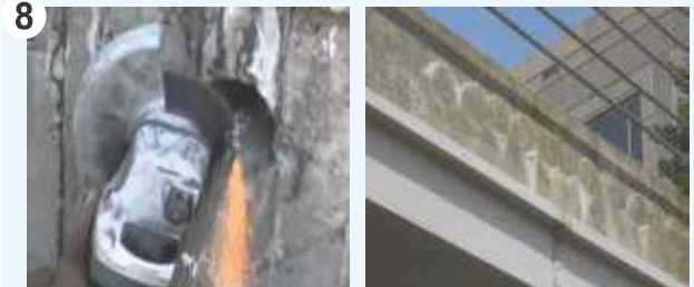
CUTTING OF EXCESS CABLE & POCKET FILLING
