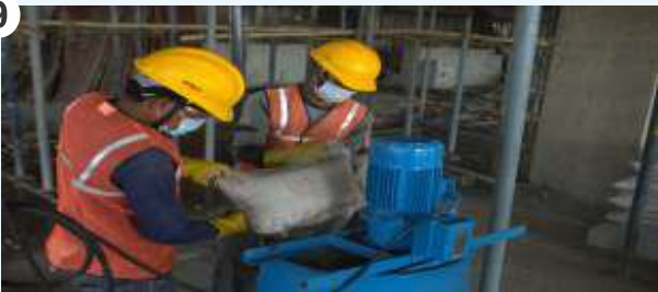
GROUTING (IN CASE OF BONDED SYSTEM)
