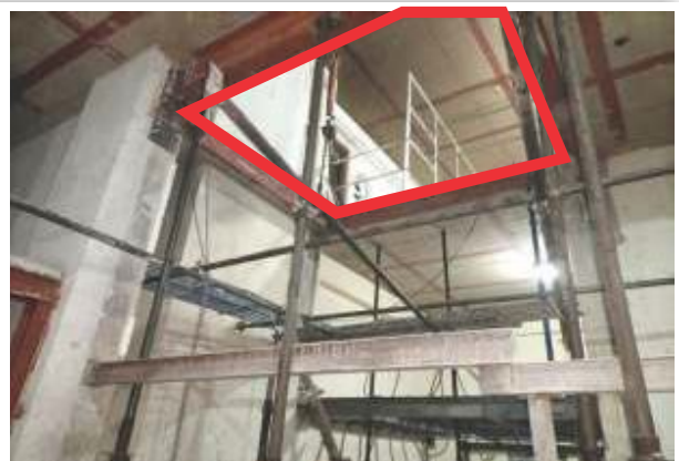
6.CUT PIECE REMOVED
