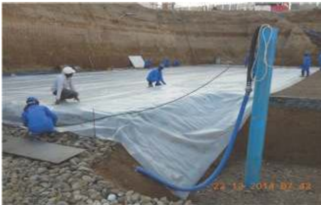
3. PLASTIC SHEET PLACING
