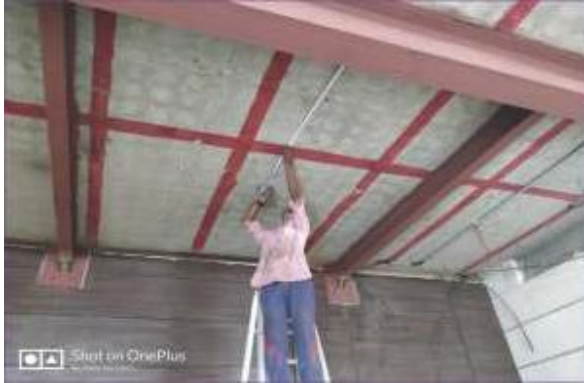
1.SLAB STRENGTHENING
