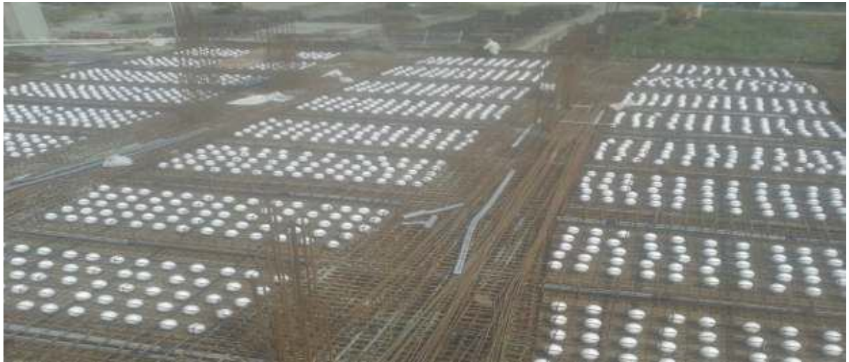
VOIDED PT SLAB CONSTRUCTION PHOTOS
