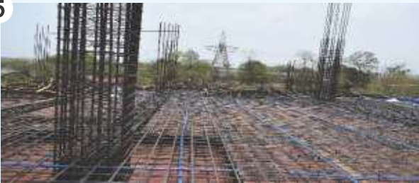
TOP REINFORCEMENT
