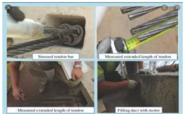
6. STRESSING & GROUTING
